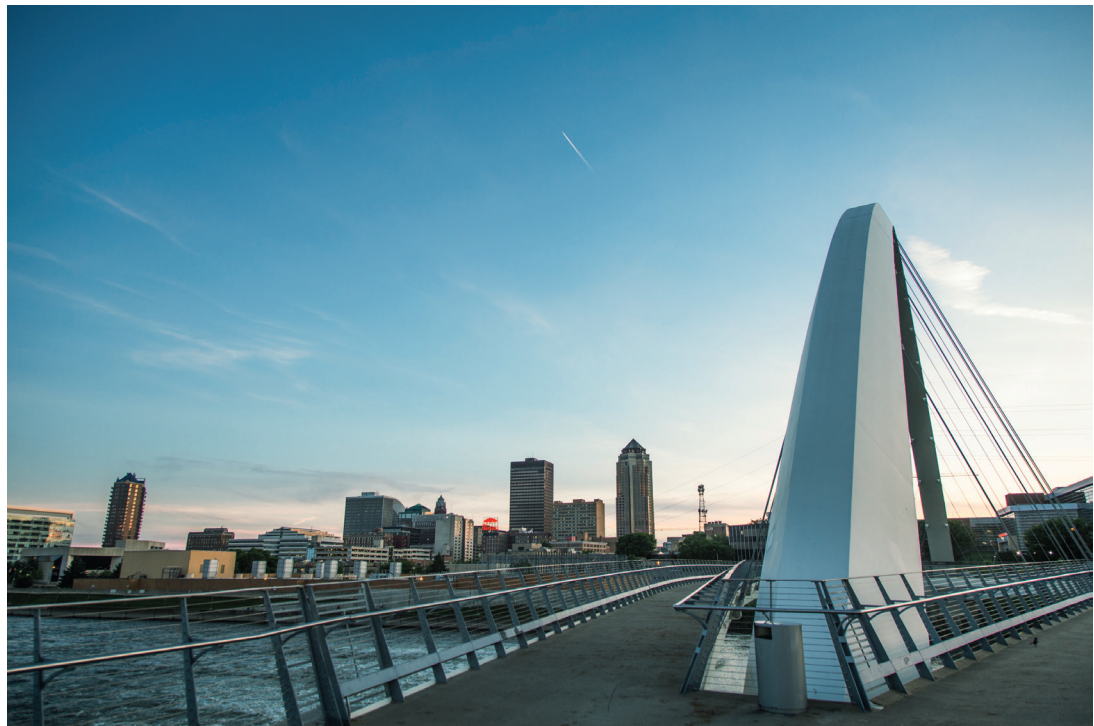
Figure 5: Pedestrian bridge over the Des Moines River
